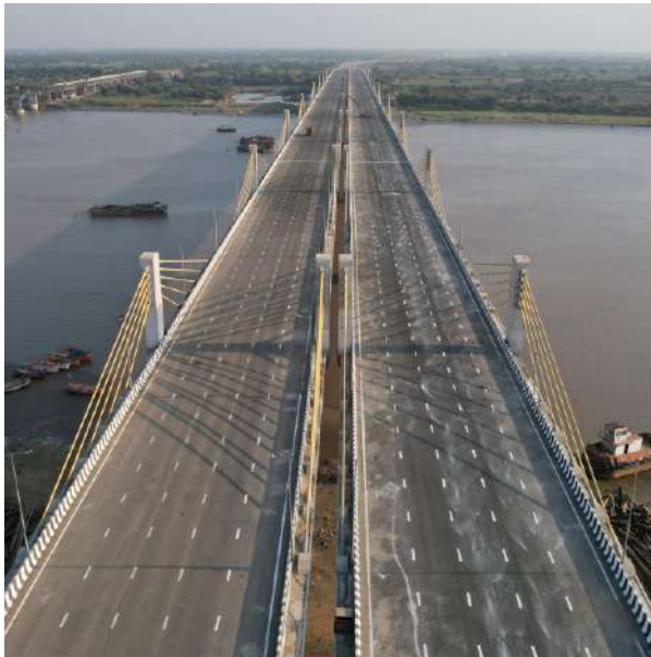
India's First 8 lane Extra Dosed Cable Stayed Bridge Across River Narmada
