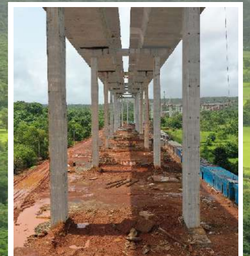
The elevated corridor consists of numerous piers that reach height of up to 40 meters.
